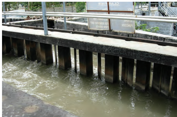
Fig. 13.4 Grit and sand removal tank
